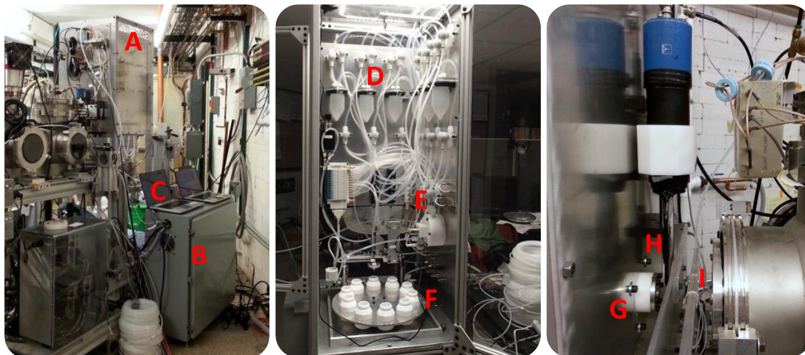
Figure 3-3. Photographs of the water cell collection end-station. (Left) Installation in the vault where the beam enters from the left, A is the side of the isolation box that holds the target cell and associated plumbing (see Fig. 3-2). B houses the electronic controls and C is a laptop that controls the system. (Center) Side view of the target end-station that shows D : the water reservoir system, E : the PTFE target cell and F : the rotating collection bottle system, (Right) Close up of the end of the beam line and G : water cell window, H : a removable scintillator in front of the target assembly, I : beam collimator.
