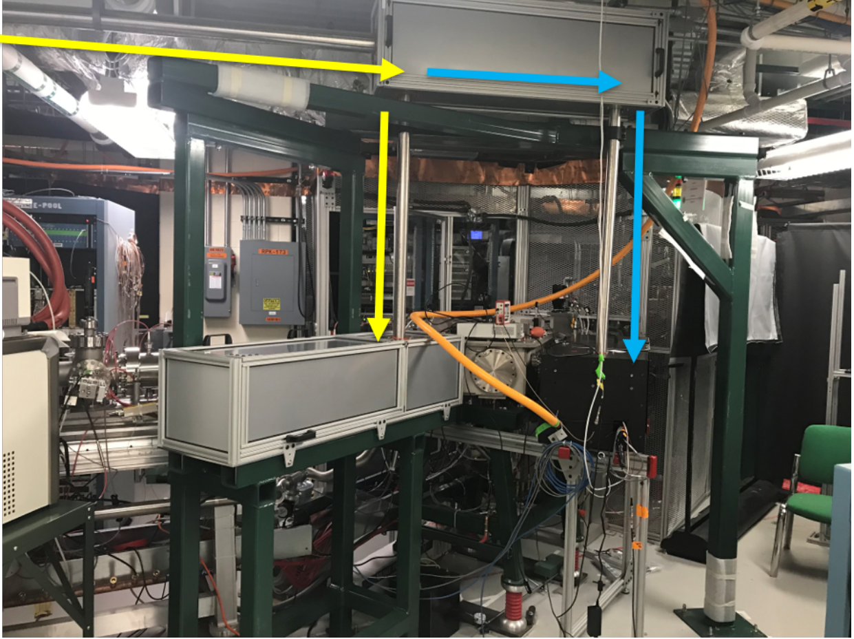
Figure 4.23: New laser safety boxes constructed in the BECOLA experimental area. Laser light from the BECOLA laser room is sent through a 10-m long steel pipe to the laser boxes. The upper box contains two breadboards to direct the light through steel pipes to the lower boxes for preparation before injection into the CLS beamline and RFQ ion trap.
